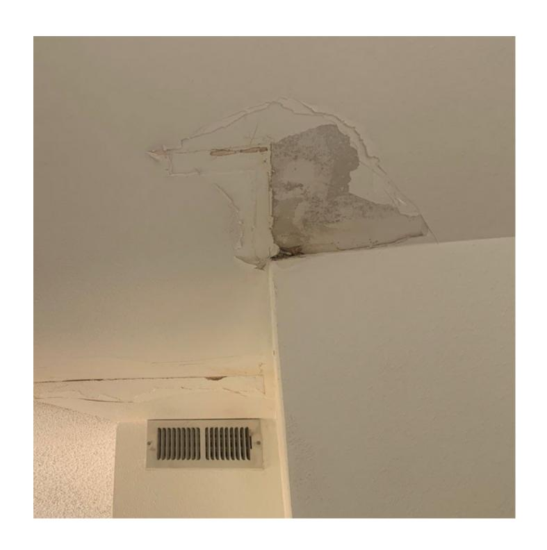
Interior water damage caused by a roof leak looks different than damage caused by pipe leaks. Determining whether the internal water damage is from your roof can be relatively simple. Water damage from a roof leak most often occurs at the lowest point of your roof. The lowest point is often in a valley at the eave of your roof.
