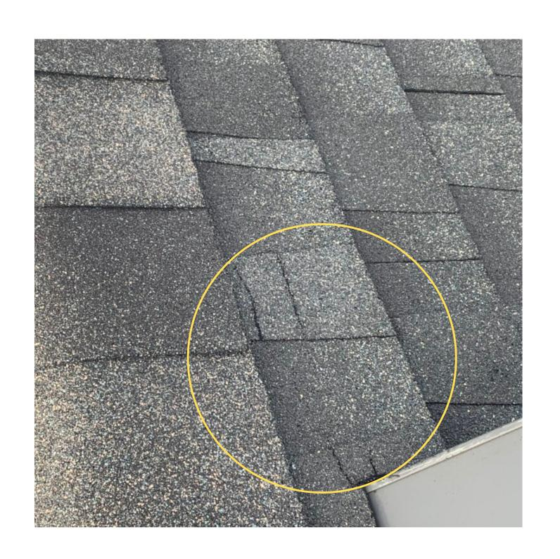
Weather damage occurs after severe weather events like a heavy wind or hail storm. Damaged shingles from a previous weather event leaves you more susceptible to weather damage moving forward. For example, wind-damaged shingles that are cracked or torn will be more likely to fail and cause leaks or damage to your underlayment. That damage to your underlayment can compromise your entire roofing system over time and could cost a great deal of money to repair if left unattended.
