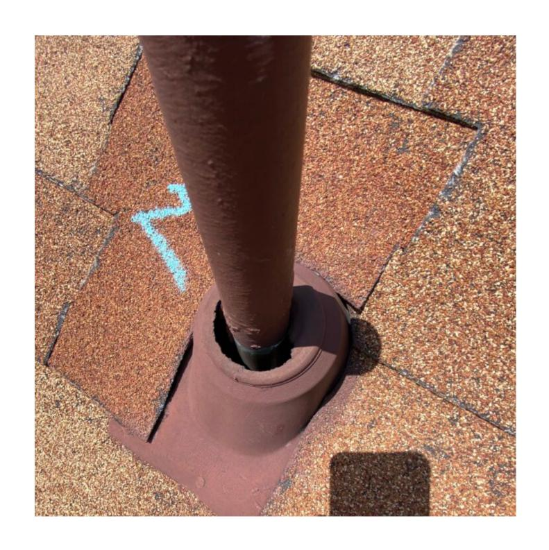
Leaks are often caused by damaged roof seals or damaged shingles. Leaks can be very obvious (with water coming into your home) or not obvious at all. Your roof might be leaking, and you don't even know it. Water can slowly seep into your decking or insulation and may not show for a long time. By the time you notice a leak, the damage done may be more extensive than what you can see.
